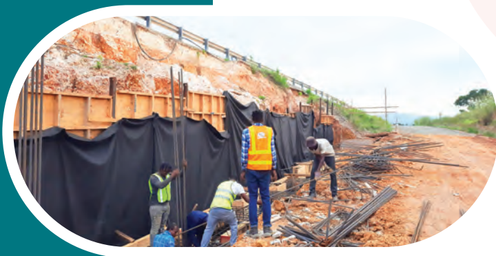
Figure 1.3: The construction of a new retaining wall along the northbound leg of the North-South Toll Road.
