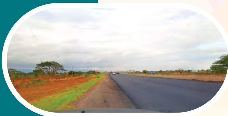
Figure 1.4: Road markings being installed along a freshly paved section along the roadway of the East-West Toll Road.
