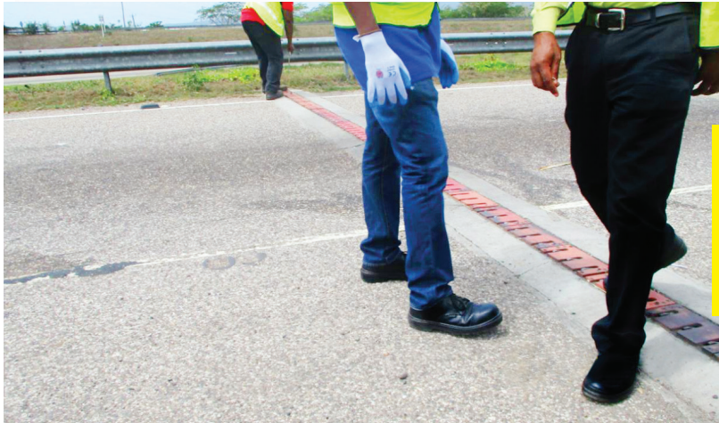
FIGURE 2:0: Shows tyre shredders being checked to ensure that they were in proper working order. This has to be done on a bi-annual basis before recertification by the Toll Authority.
