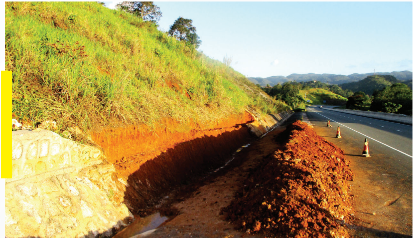
FIGURE 1.5: Above shows the reconstruction of a V-drain along the roadway. V-drains facilitate adequate drainage of the roadway.
