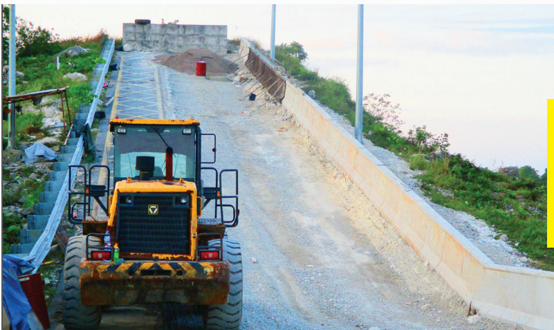
FIGURE 1.6: Above shows the reconstruction of one of the Escape Lanes along the northbound leg of the toll road. These escape lanes were designed to facilitate runaway vehicles.
