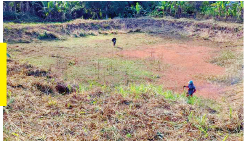
FIGURE 1:8: Above shows the removal of excess vegetation from an infiltration pond along the northbound leg of the toll road. Infiltration ponds significantly reduce the likelihood of flooding of nearby communities.
