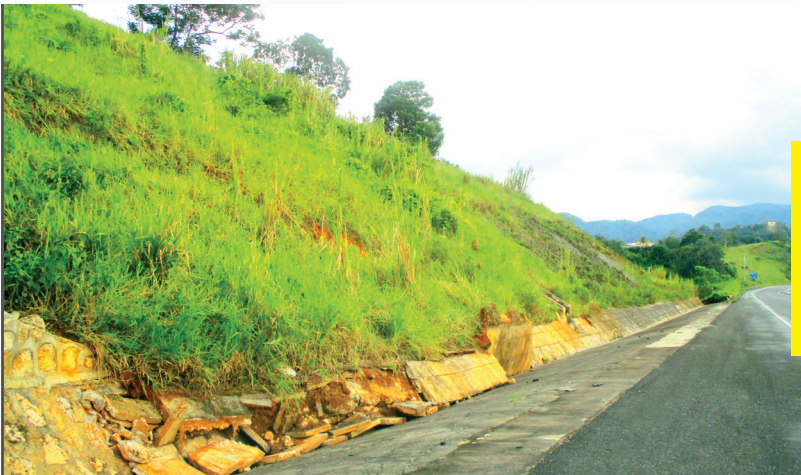
FIGURE 1.5: Above shows the reconstruction of a V-drain along the roadway. V-drains facilitate adequate drainage of the roadway.
