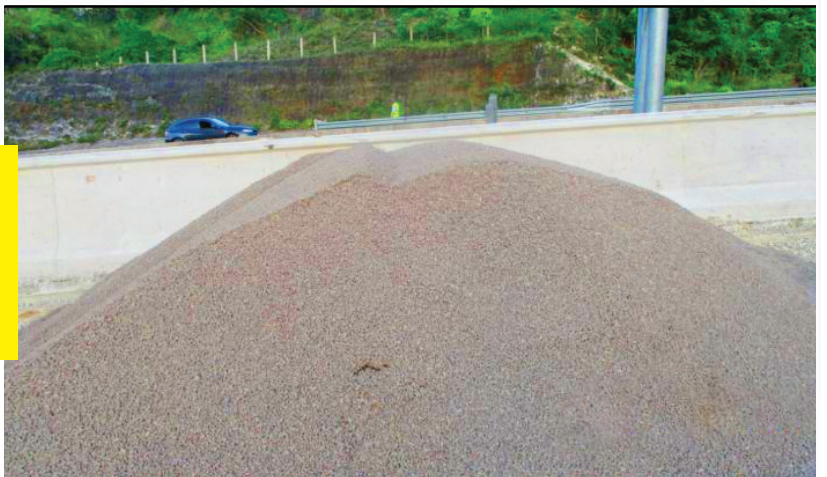
FIGURE 1.6: Above shows the reconstruction of one of the Escape Lanes along the northbound leg of the toll road. These escape lanes were designed to facilitate runaway vehicles.
