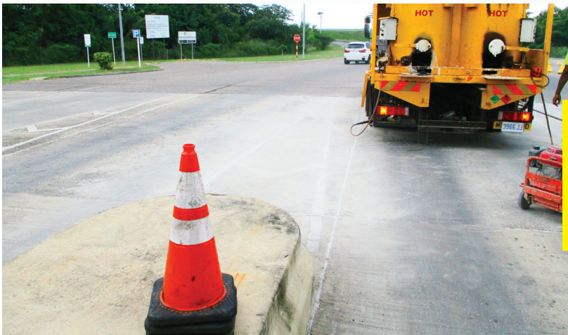
Figure 1:9: Above shows road marking being conducted at one of the toll plazas.
