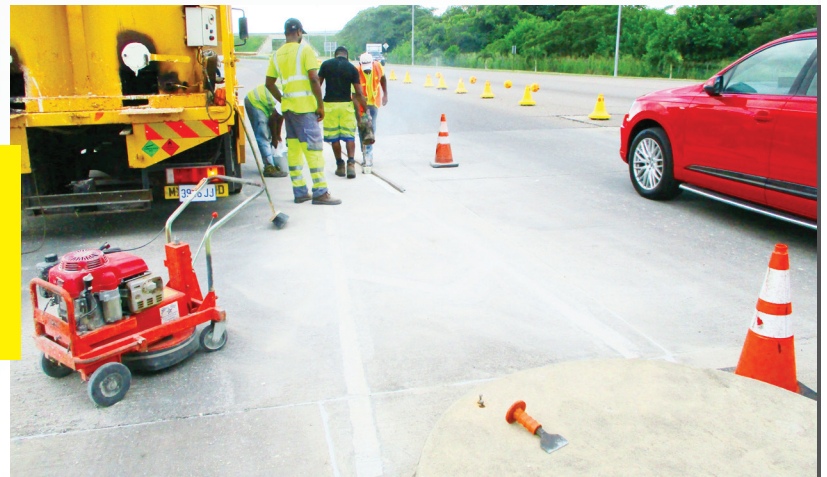
Figure 1:9: Above shows road marking being conducted at one of the toll plazas.
