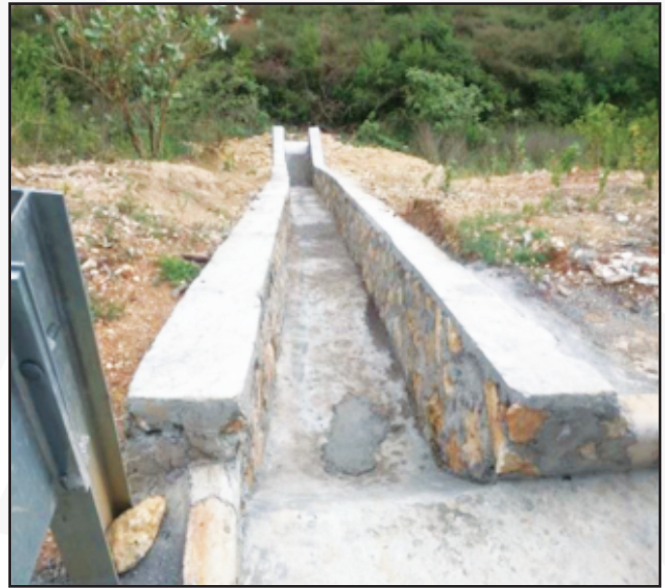
Figure 1.8 Above shows water ponding on the North-South Highway (left) and the completed chute drain constructed to alleviate this issue (right). Water that settles on the toll road creates an environment for hydroplaning to occur.
