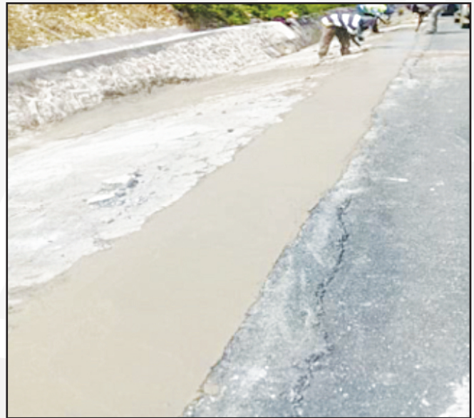
Figure 2.0 Above shows the construction of a rubble retaining wall (left) and the repair of a damaged concrete drain (right). A lane closure application and a traffic management plan were approved by the Toll Authority in relation to these works.
