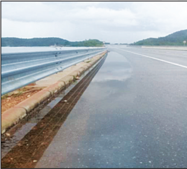
Figure 1.8 Above shows water ponding on the North-South Highway (left) and the completed chute drain constructed to alleviate this issue (right). Water that settles on the toll road creates an environment for hydroplaning to occur.
