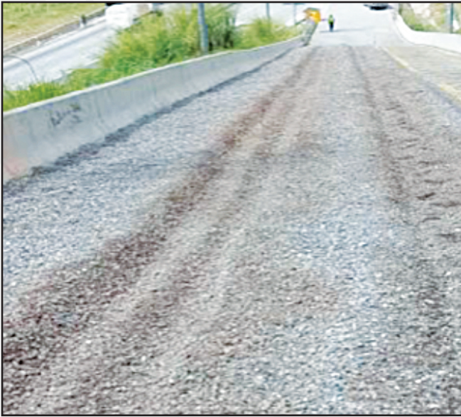
Figure 1.5 Above shows the cleaning of an escape lane on the North-South Highway to remove vegetation and faulty material. An escape lane is a traffic device that enables vehicles that are having braking problems to safely stop. Vegetation and faulty material reduce the effectiveness of the gravel to allow a vehicle's momentum to be dissipated in a controlled way. A lane closure application and a traffic management plan were submitted to the Toll Authority for review and approval; repairs lasted for 72 hours or more.
