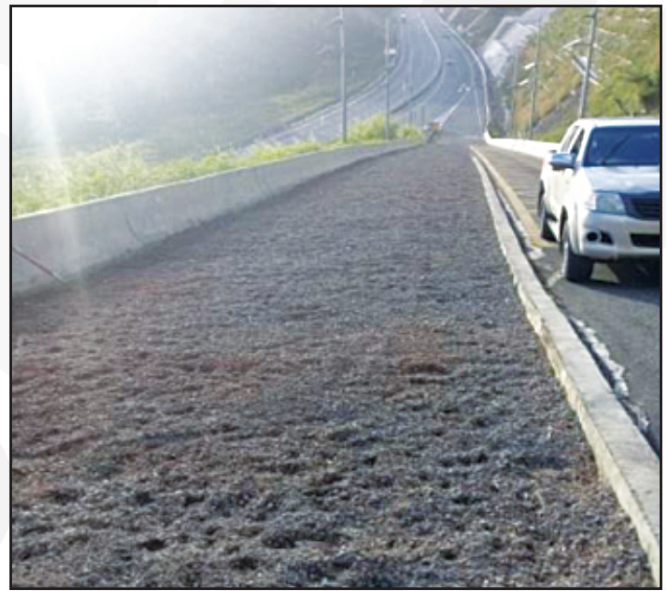
Figure 2.1 Shows before and after images of an escape lane on the North-South Highway. The before image shows vegetation growing in the arrestor bed and the other image was taken after maintenance works were completed.
