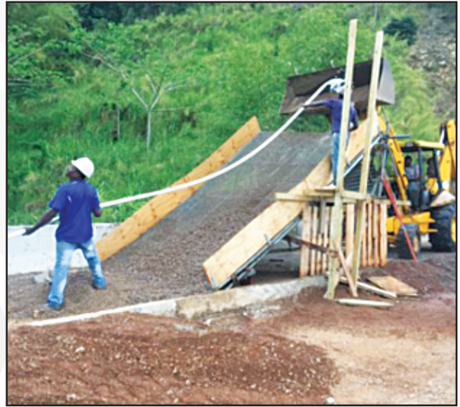
Figure 1.5 Above shows the cleaning of an escape lane on the North-South Highway to remove vegetation and faulty material. An escape lane is a traffic device that enables vehicles that are having braking problems to safely stop. Vegetation and faulty material reduce the effectiveness of the gravel to allow a vehicle's momentum to be dissipated in a controlled way. A lane closure application and a traffic management plan were submitted to the Toll Authority for review and approval; repairs lasted for 72 hours or more.
