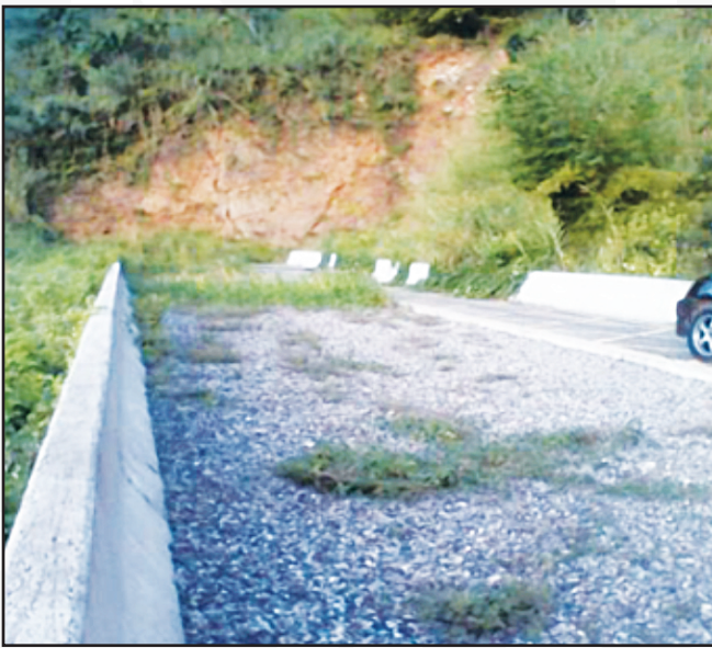
Figure 2.1 Shows before and after images of an escape lane on the North-South Highway. The before image shows vegetation growing in the arrestor bed and the other image was taken after maintenance works were completed.
