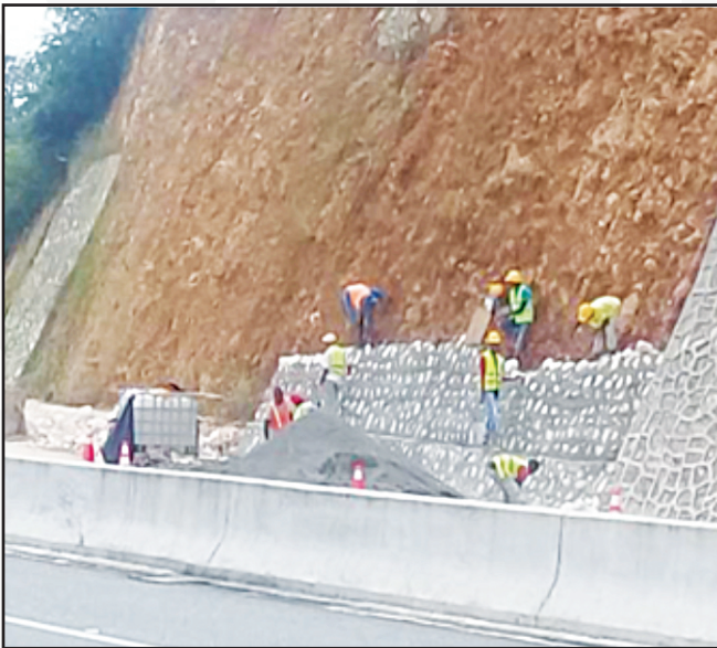
Figure 2.0 Above shows the construction of a rubble retaining wall (left) and the repair of a damaged concrete drain (right). A lane closure application and a traffic management plan were approved by the Toll Authority in relation to these works.
