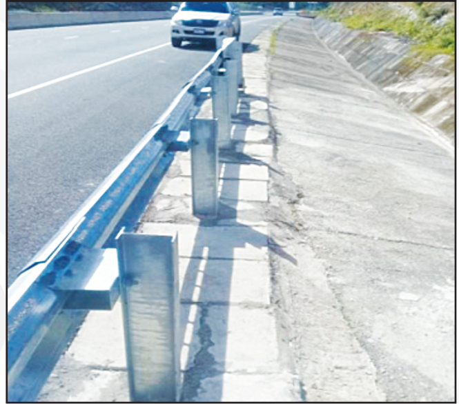
Figure 1.9 Above shows repair work done on a damaged guardrail of the North-South Highway. Repair work for damaged guardrails is an ongoing activity on the North-South Highway due to the high frequency of collisions. A lane closure application and a traffic management plan were approved by the Toll Authority.
