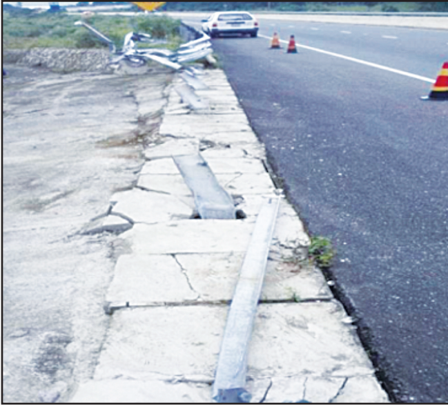
Figure 1.9 Above shows repair work done on a damaged guardrail of the North-South Highway. Repair work for damaged guardrails is an ongoing activity on the North-South Highway due to the high frequency of collisions. A lane closure application and a traffic management plan were approved by the Toll Authority.
